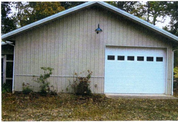
30' X 40' Metal Building
